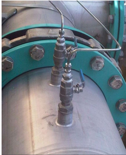
Figure 7 - Ball valve assembly
